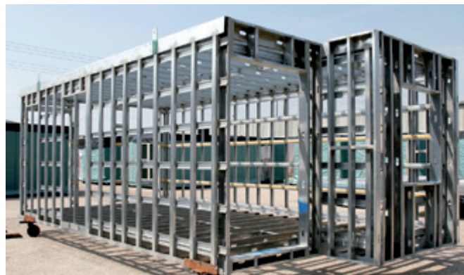
Figure 1 Four sided module (with staggered end) (Image courtesy of Ayrshire Framing)
