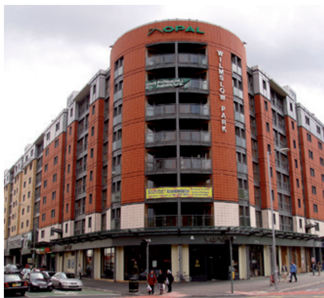
Figure 8 Podium structure used to support residential modular units (Image courtesy of The Design Bureau and Ayrshire Framing)
