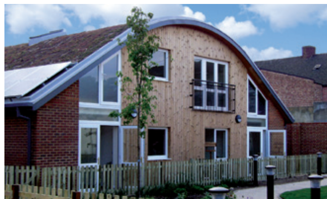
Figure 15 Light steel energy efficient housing constructed using modules (Image courtesy of Ayrshire Metal and Futureform)
