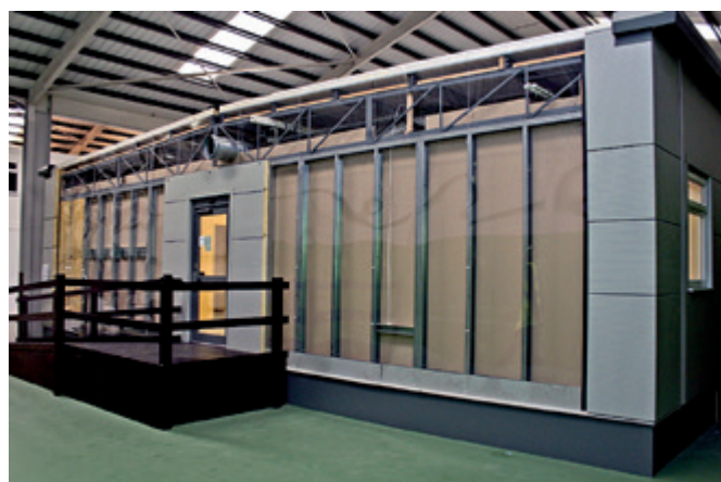
Figure 5 Demonstration modular hospital ward building (with perspex wall to show construction) (Image courtesy of BW Industries)
