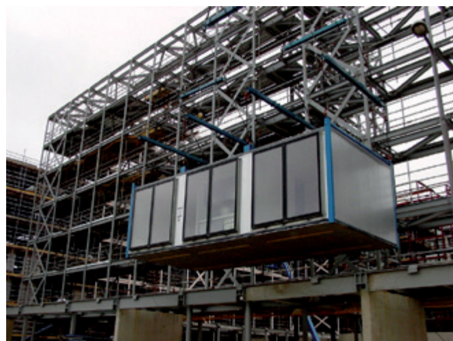
Figure 9 Installation of modules behind external steel framework at MoHo, Manchester (Image courtesy of Yorkon and Joule Consulting Engineers)
