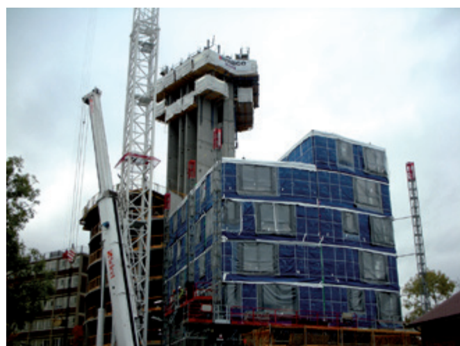
Figure 10 Concrete core used to stabilise 16 storeys of modules (Image courtesy of Futureform and Ayrshire Framing)
