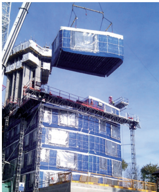
Figure 3 Partially open sided modules (Image courtesy of Futureform and Ayrshire Framing)
