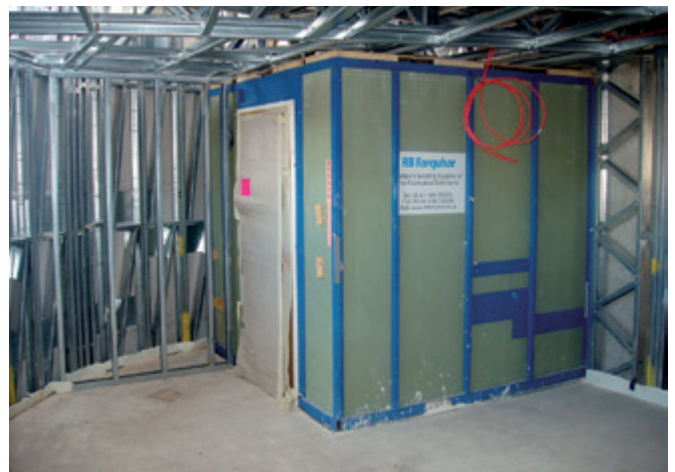
Figure 12 Toilet pod used with light steel framing in a hotel (Image courtesy of Metek UK)
