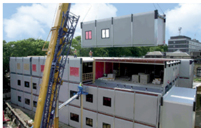
Figure 7 Installation of open sided modules for a hospital (Image courtesy of Yorkon)
