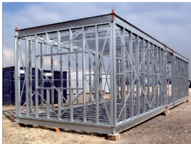
Figure 2 Long four-sided module with an integral corridor (Image courtesy of Kingspan)
