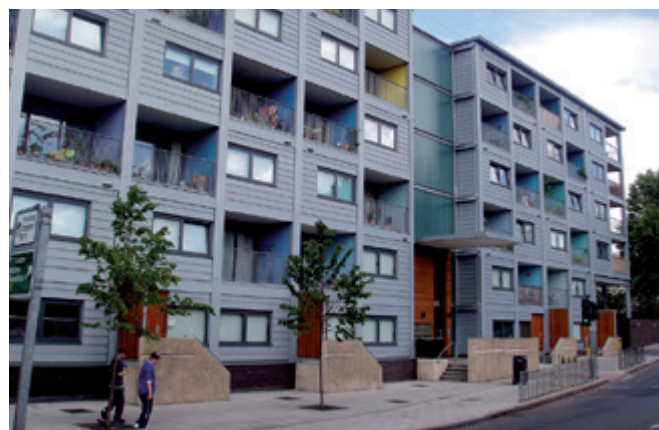
Figure 14 Raines Court, London showing modular construction with integral balconies (Image courtesy of Alford Hall Monaghan Morris and Yorkon)
